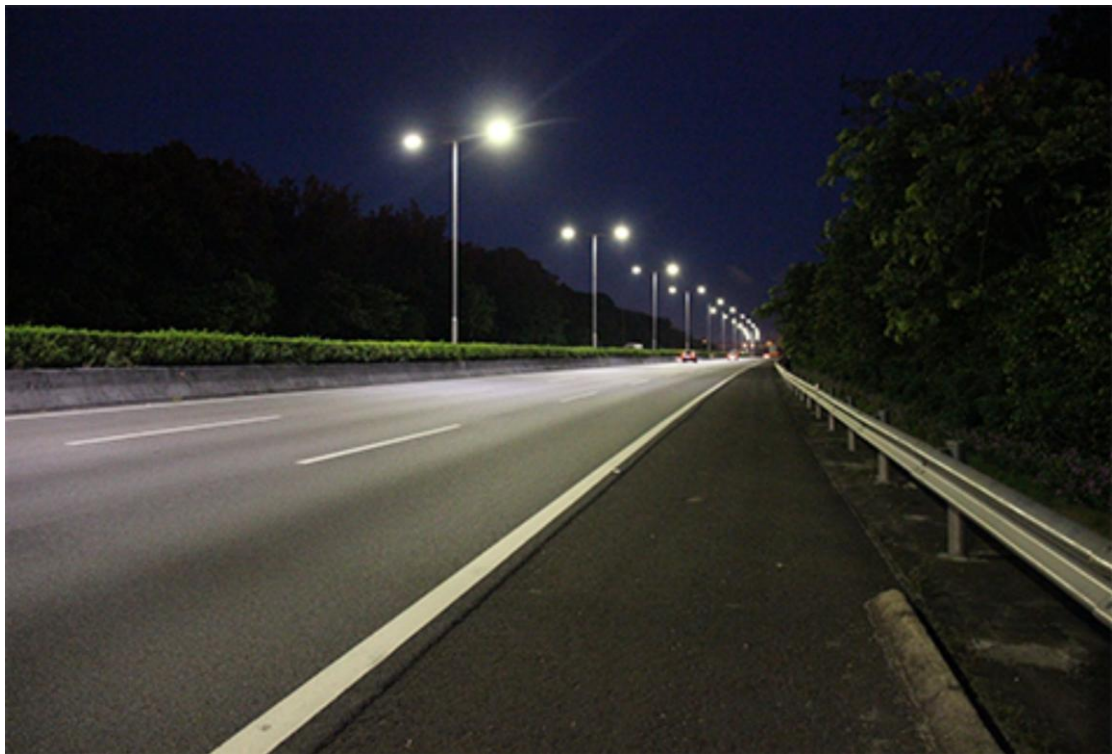
Guangzhou-Shenzhen Expressway Road Lamp Reconstruction Project
