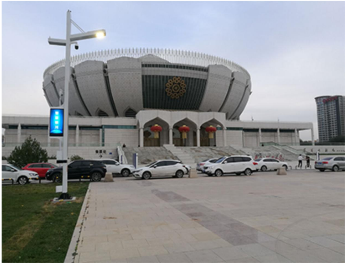
Yinchuan intelligent streetlight project
