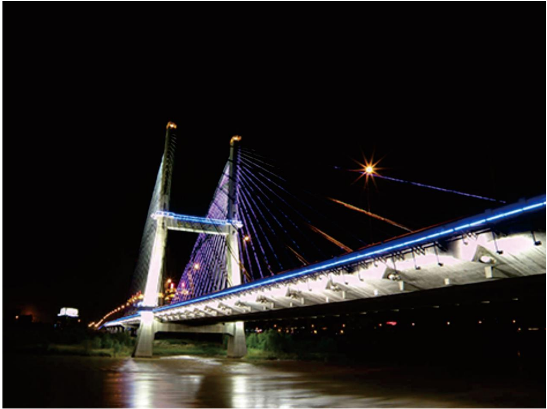
Renovation of lighting project of Huanghe River Bridge in Lanzhou
