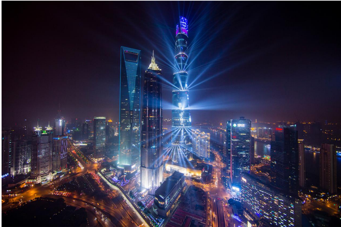
Lighting project of Shanghai Center Building
